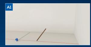
Prime the surface and level if necessary Mix tile adhesive Mark the installation area Cut sheeting and sealing tapes to size
