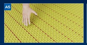
Lay the heating cables according to your individual requirements. Follow the manufacturer's instructions for installation and connection!
