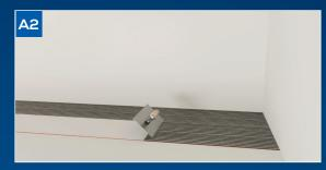
Apply tile adhesive to the surface with a 6 x 6 mm notched trowel.
